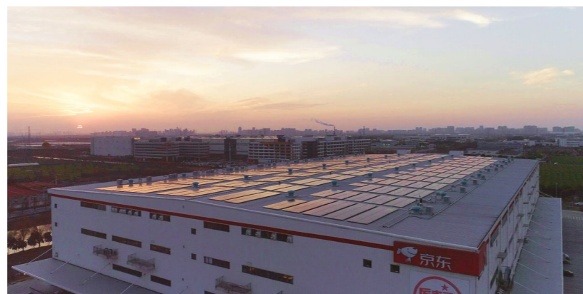
Distributed Photovoltaic Roof
